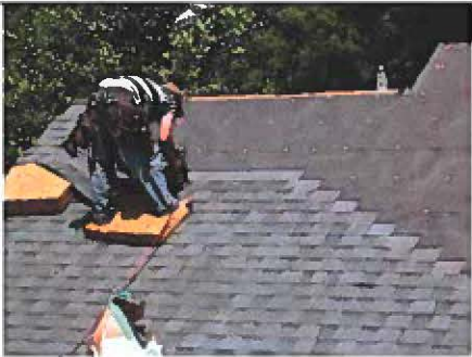
Replacement of roofing in Virginia Beach
