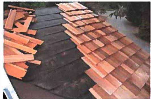
Replacement of roofing in Leesburg
